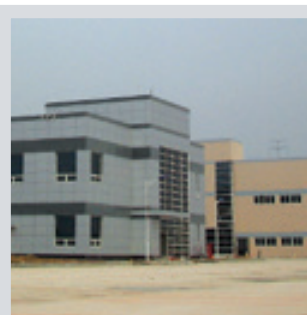
Wuxi Plant (China)
